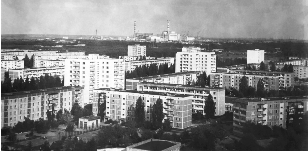
1 The city of Prip'yat in the early 80s, with the Chernobyl Atomic Energy Station visible on the horizon. Reactor Unit Four of the plant lay just three kilometers from the southeastern edge of the town.
