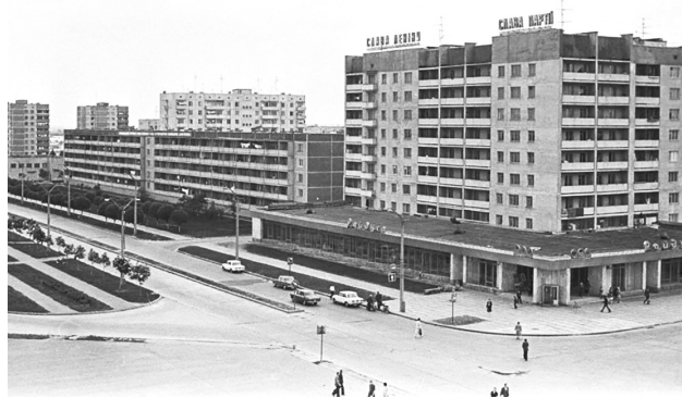
3 The Raduga—or Rainbow—department store on the corner of Kurchatov Street and the end of Lenina Prospekt. Plant director Viktor Brukhanov, like other senior members of the station staff, lived in an apartment above the store. The letters on the rooftop read “Glory to Lenin!” and “Glory to the Party!”
