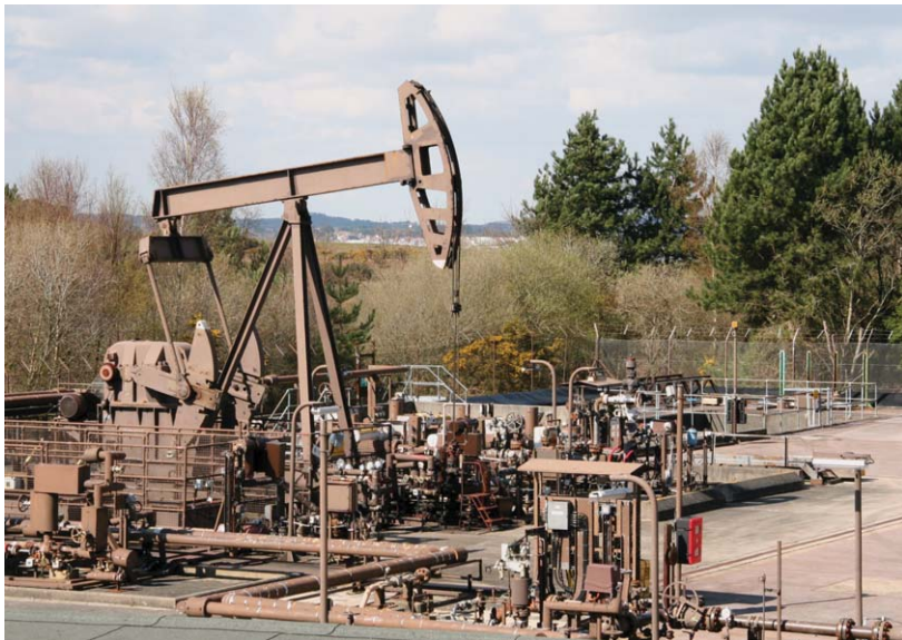
Figure 6.39 Rod pump and compact pad.
