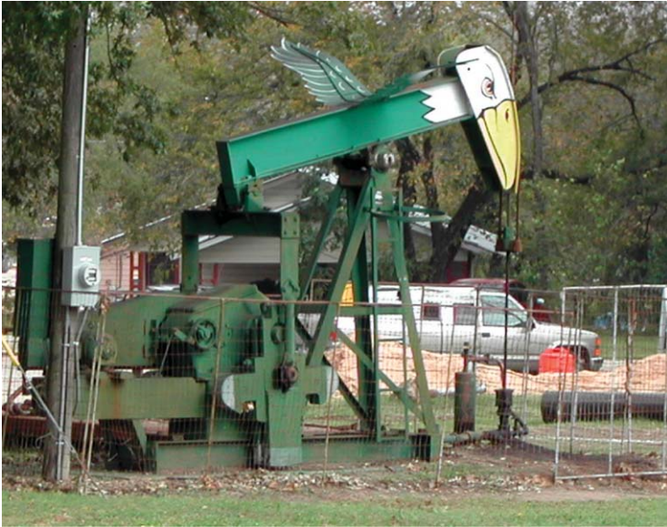
Figure 6.38 Rod pump in children's play park.
