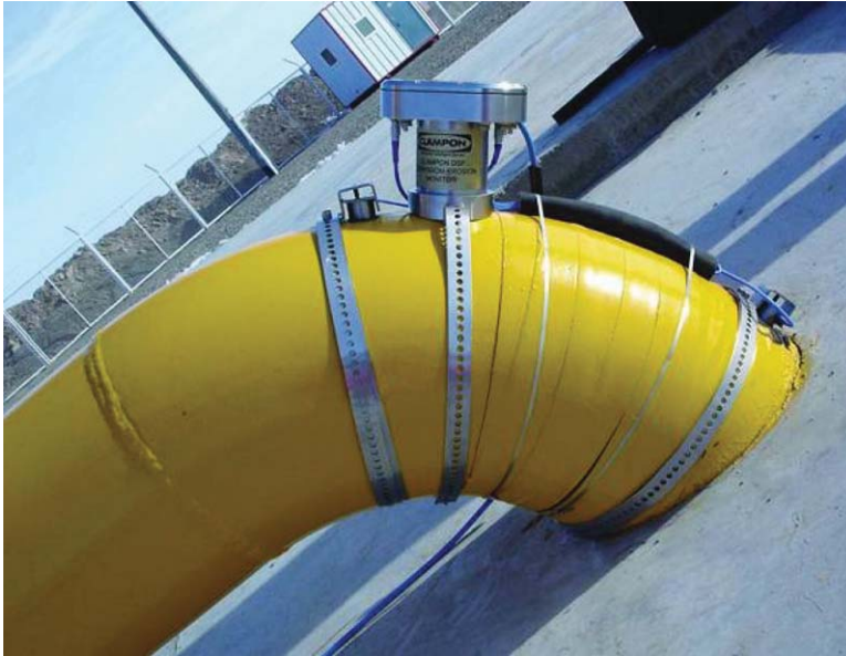
Figure 3.23 Ultrasonic sand detector incorporating an erosion and corrosion monitor. Source: Photograph courtesy of ClampOn Inc.
