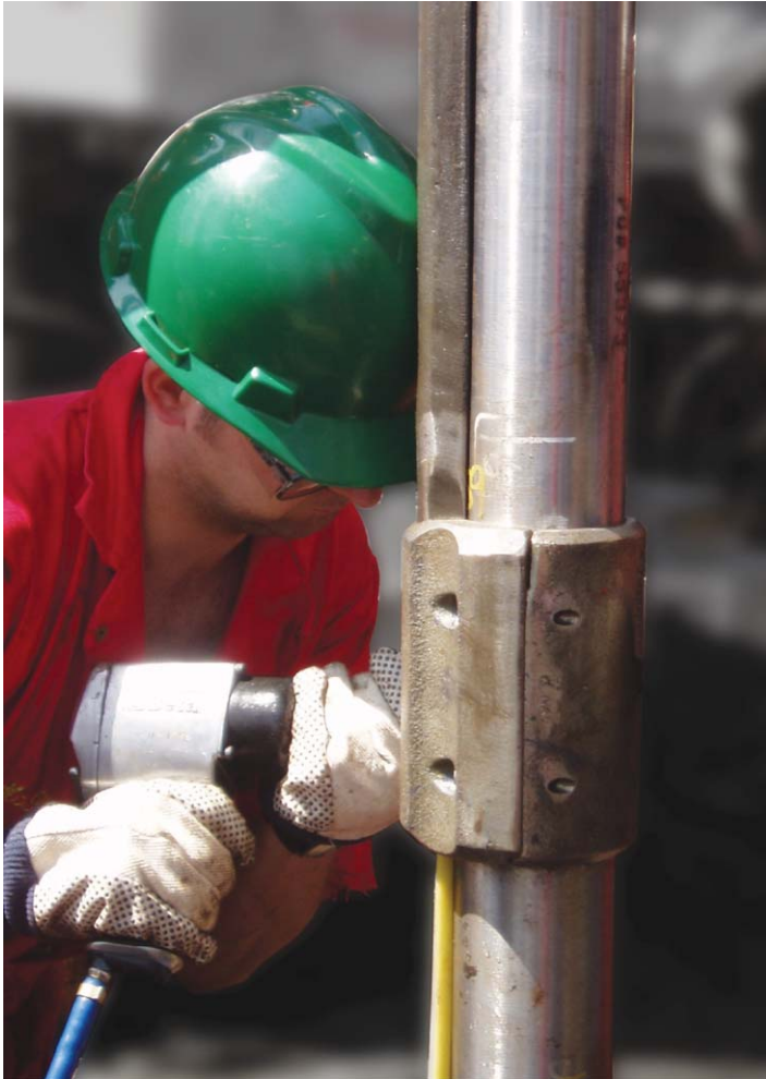
Figure 12.16 Installing a control line protection plate.
