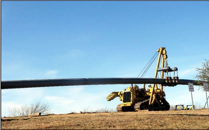
FIGURE 15.1 Installing onshore pipelines. (Source: © energy.fanchi.com (2010).)
