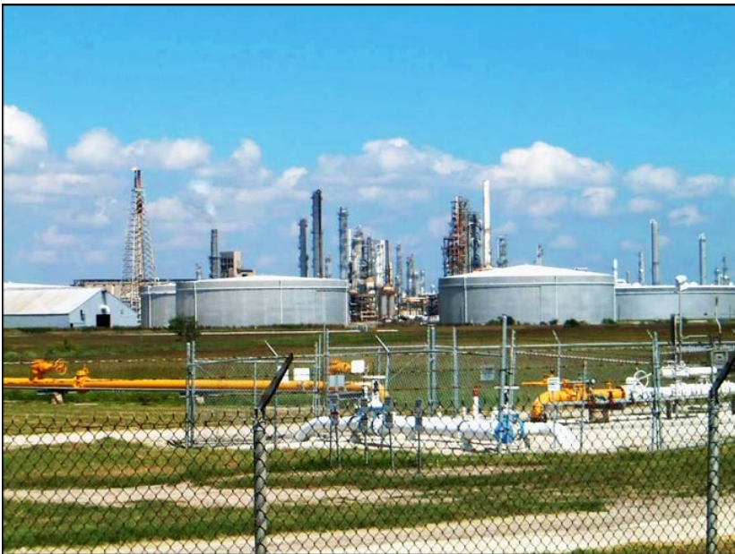
FIGURE 15.3 South Texas refinery. (Source: © energy.fanchi.com (2002).)
