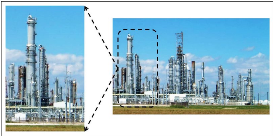
FIGURE 15.4 Distillation towers at a Texas refinery. (Source: © energy.fanchi.com (2015).)
