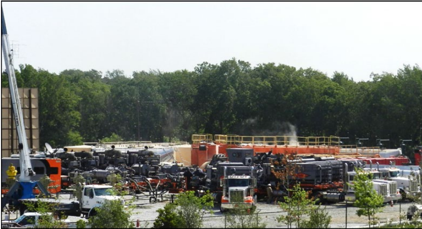
FIGURE 10.2 Hydraulic fracturing operation in Mansfield, Texas.
