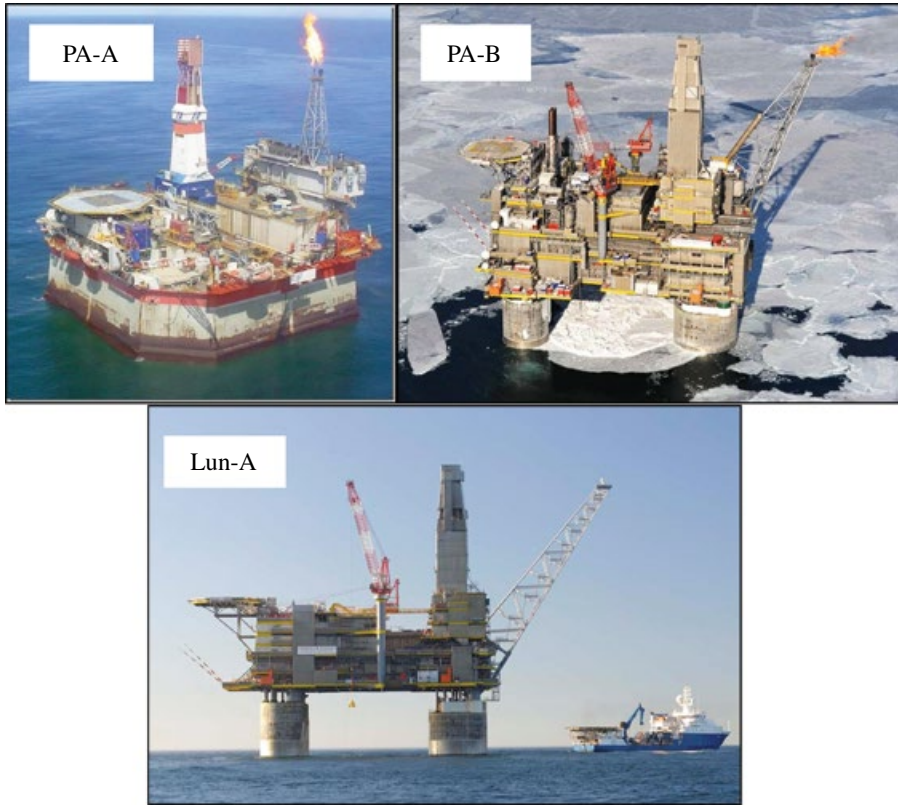
FIGURE 15.10 PA-A (Molikpaq) platform, PA-B platform, and Lun-A platform. (Source: Courtesy of Sakhalin Energy (2016), personal communication.)
