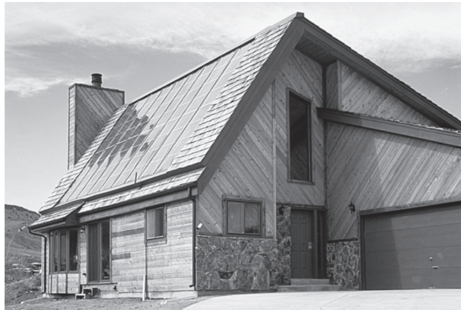
Figure 13.24 This home in Golden, Colorado uses a liquid-based solar system for space and water heating. Source: Courtesy of DOE/NREL
